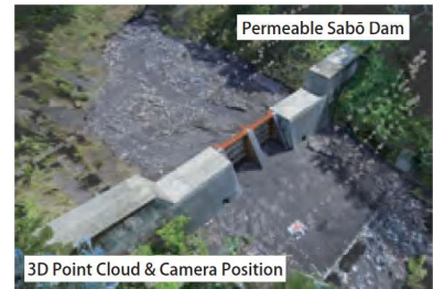
Detailed inspection using a UAV equipped with Visual SLAM
