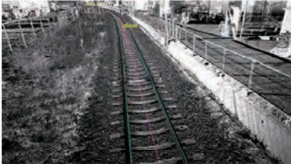
Automated extraction of railway features from laser point clouds using RaiLis
