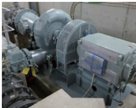
Small Hydroelectric Power Generation (Magoishi hydroelectric power plant /Aqua Power Tohoku Co.,Ltd)
