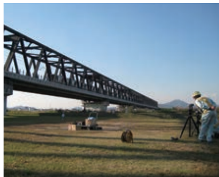
Bridge Deflection Measurement System
